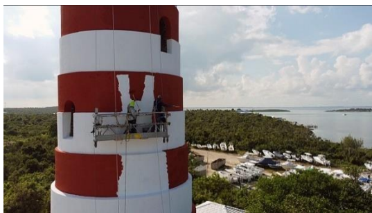
Work in Progress on the Tower Repair
