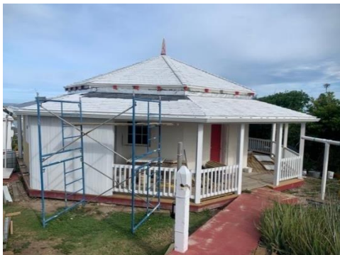
Repairs underway for the Keeper's House
