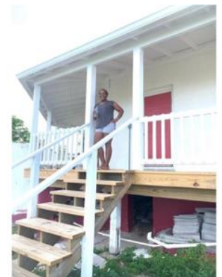
The Assistant Keeper's Family is happy to have the repairs.
