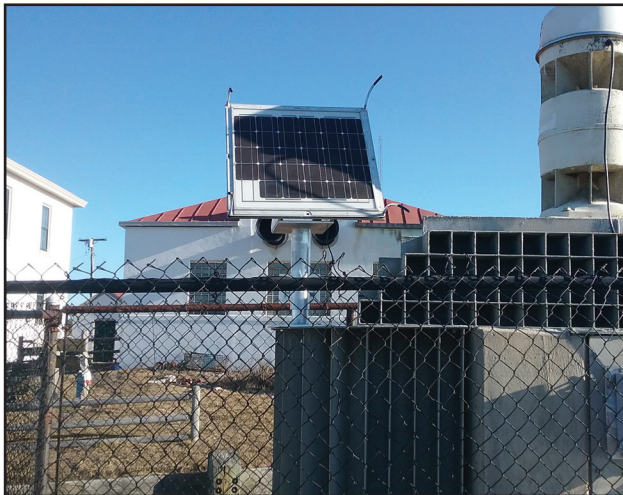
New solar panel
