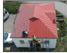
Fog Signal building during roof replacement
