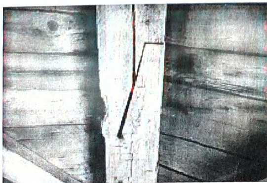
Vertical Scarf Joint
