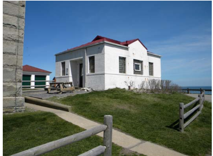
Once completed, the exterior of all buildings of the light station will have been renewed. It is one of the most photographed light station facilities on the east coast.
